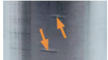
Figure 11 Raceways and rolling elements can incur indentations and nicks caused by hard, possibly sharp, objects.
